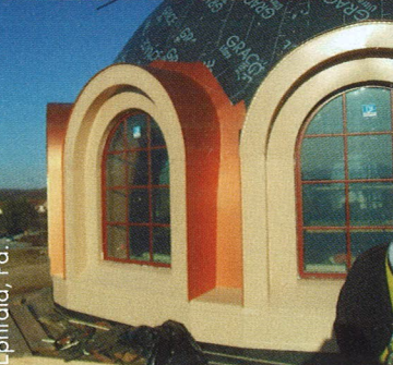
Photos courtesy of GSM Roofing, Ephrata, Pa.
