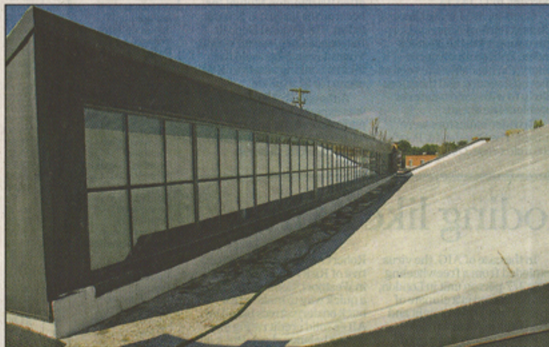
The white surface on the bank's sawtooth roof is angled toward each bank of windows.
